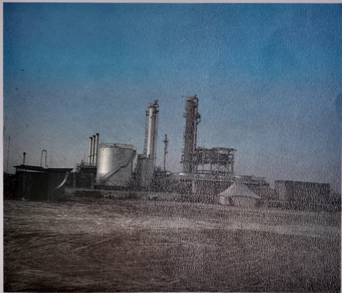
Oil installations in Abu Dhabi
