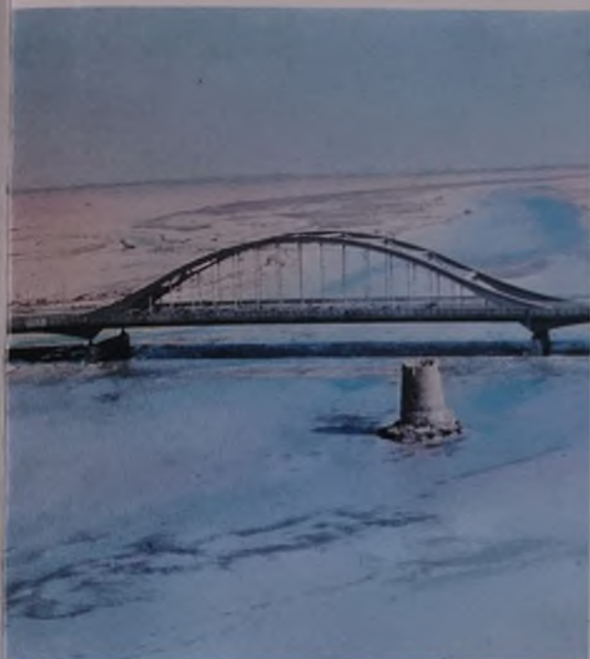
The Maktaa bridge
