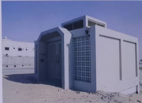
Indoor type distribution substation
