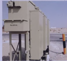
Oil Disconnect Switches - 13.8 KV
