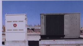
Unit Substation
