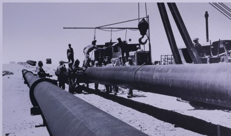
Building the Khursaniyah-Ras Tanura No. 2 pipeline.
