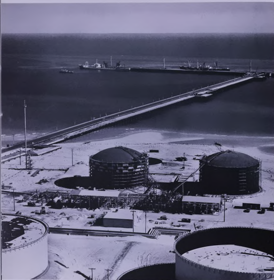
The Refrigerated LPG Plant rising near the Marine Terminal.
