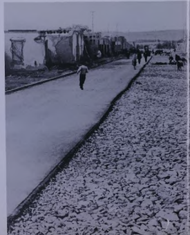
Preparing foundations and asphaltting in Ahar
