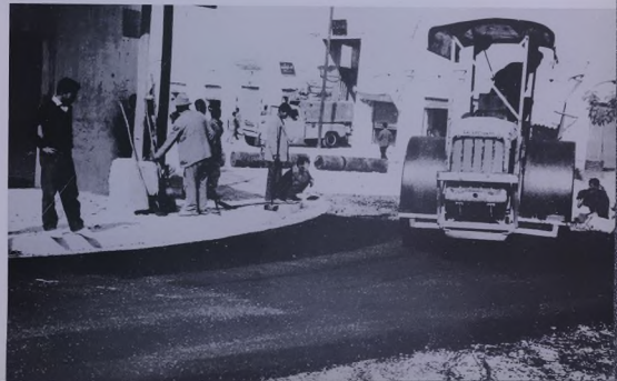
Laying asphalt in Borazjan
