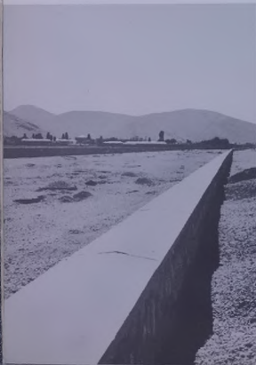
Flood control system near Shiraz
