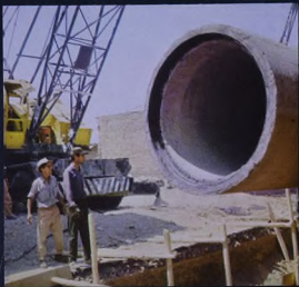
Pipelayers at work
