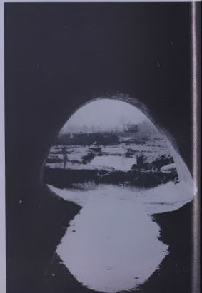
Esfahan sewerage system
