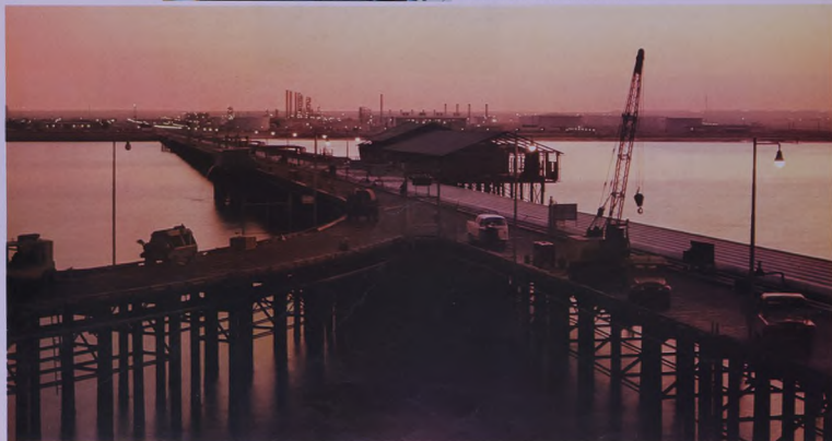
The South Pier at dusk with the refinery in the background.
