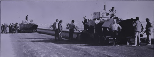
The Ahmadi-Fahahil road under construction.
