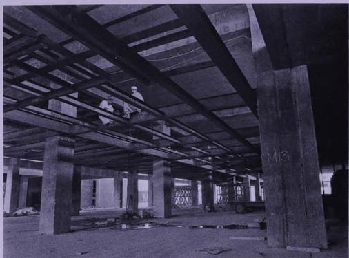
Support steelwork for AC plant and radiology equipment
