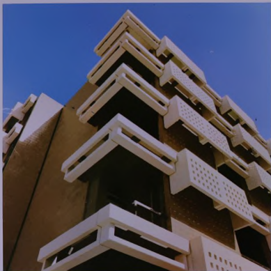
Detail of Sunbreaker units at ward balconies
