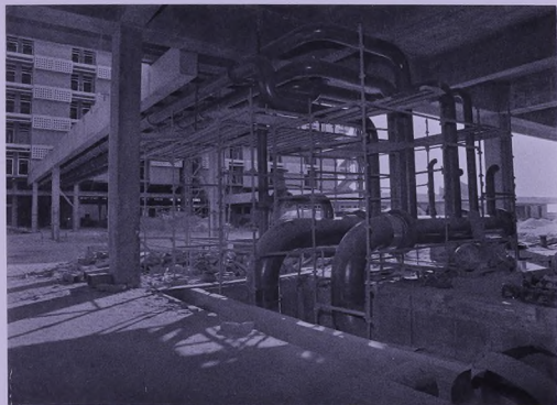
Connection of piped services to link bridge
