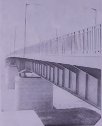
A new bridge over Diyala river
