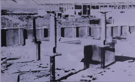
A new factory under construction in Dahok
