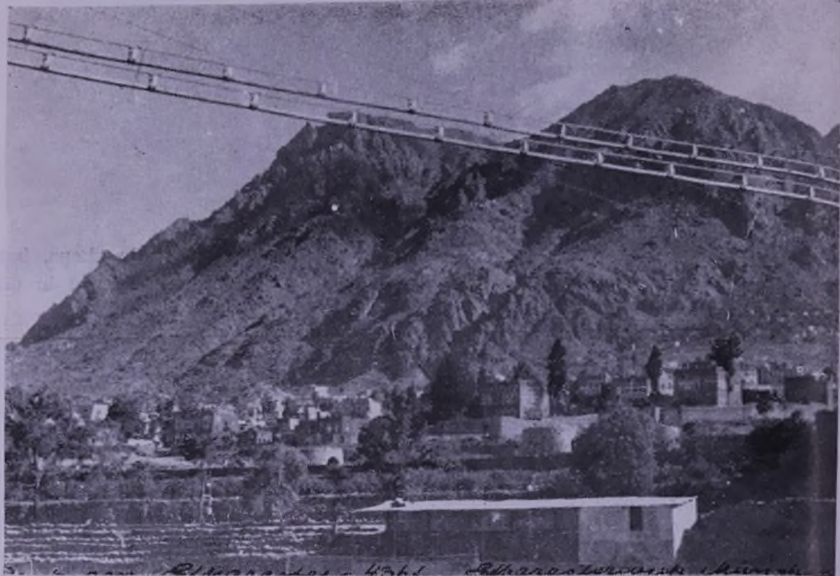
Power transmission lines across the mountains in Taz
