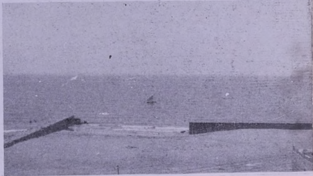
The old port of Hudaïda a picture of complete neglect
