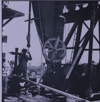
A LuFin pump being installed over the well head for testing.
