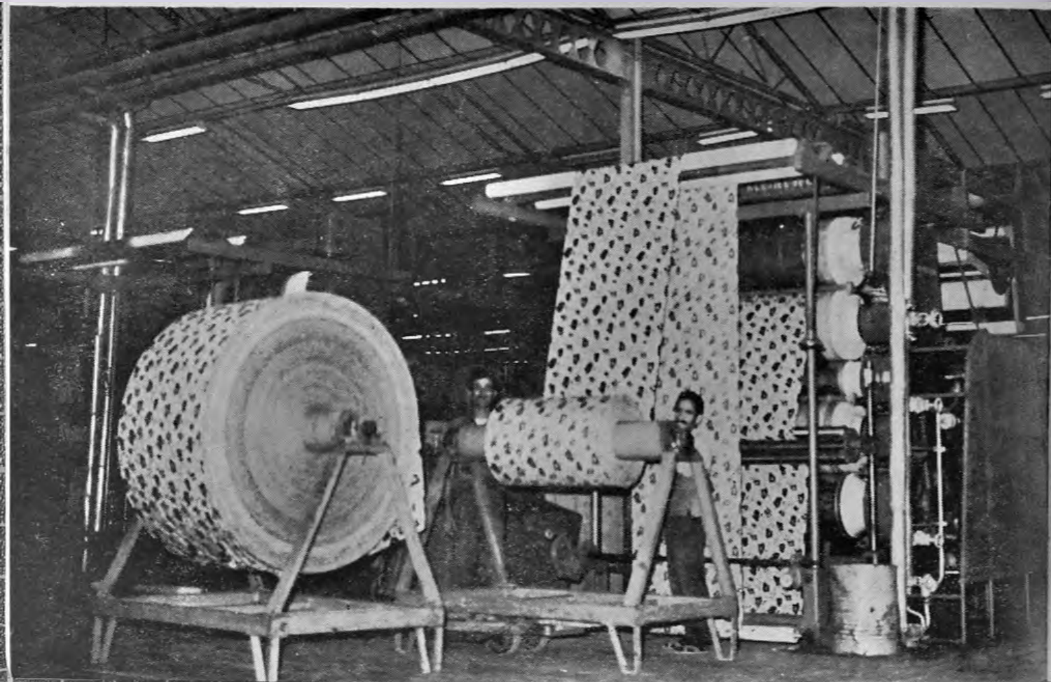
Finishing plant at Shahi No. 2 mill
