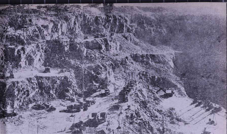
Construction of the High Dam requires the grading of hundreds of kilometres of roads, for carrying the equipment to the site.
