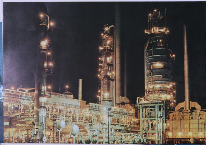
Tehran Refinery at night.
