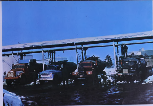
Loading road tankers
