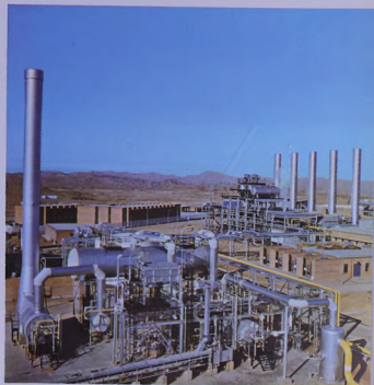
The Bak Boland Gas Refinery.
