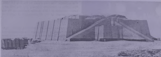
The Ziggurat after the reparation (height about 15 m.)
