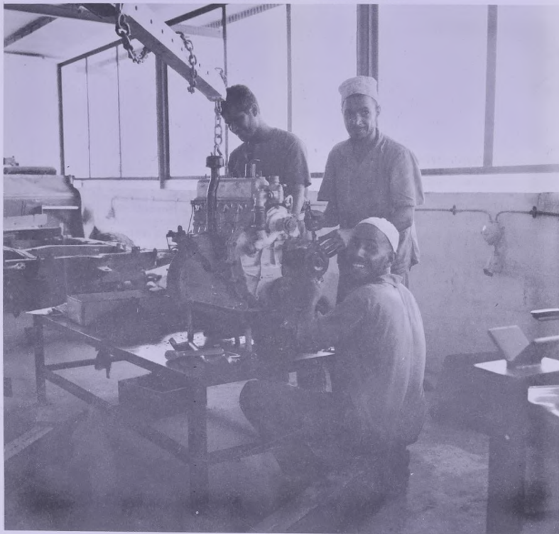
Basic automotive courses are held in a small training annexe, which has been built in the Main Workshop area. Our picture shows Sallm Ali, Said Ali and Mudhaffer Salem assembling a landrover engine.
