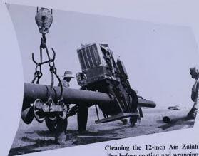
Cleaning the 12-inch Ain Zalah line before coating and wrapping
