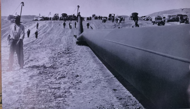
'The Third River' in its last stages of completion
