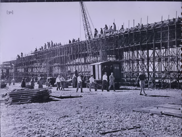
Building the Lesser Zab River Bridge
