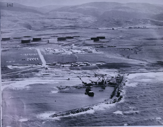
Basrah Terminal under construction
