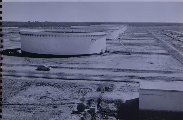
Part of the Tank Farm at Fao
