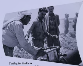
Testing for faults in the coated and wrapped line
