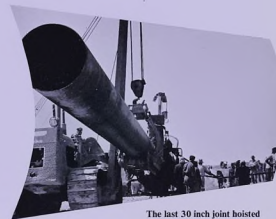
The last 30 inch joint hoisted into position before welding
