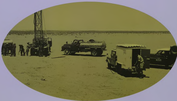
A seismic crew prepare to drill a shot hole
