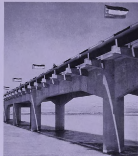
New Lesser Zab Bridge linking Baba and Acanah domes
