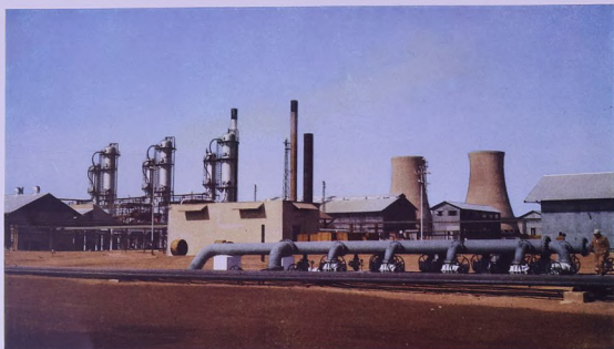
Part of the process plant at Kirkuk
