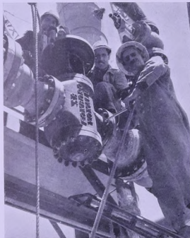
Erecting No.9 stabilisation unit
