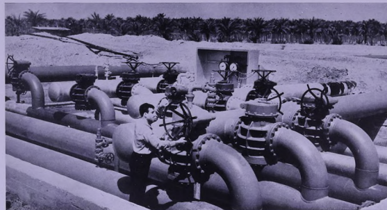
Fao terminal: the loading manifold
