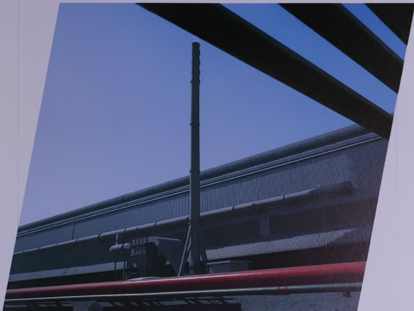
In addition to gas cleaning, which will significantly improve the environment both inside and outside the potroom, particulates of alumina will be recovered using cyclones and recycled.
