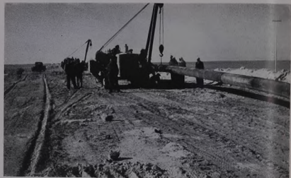
Lowering pipe into the ditch
