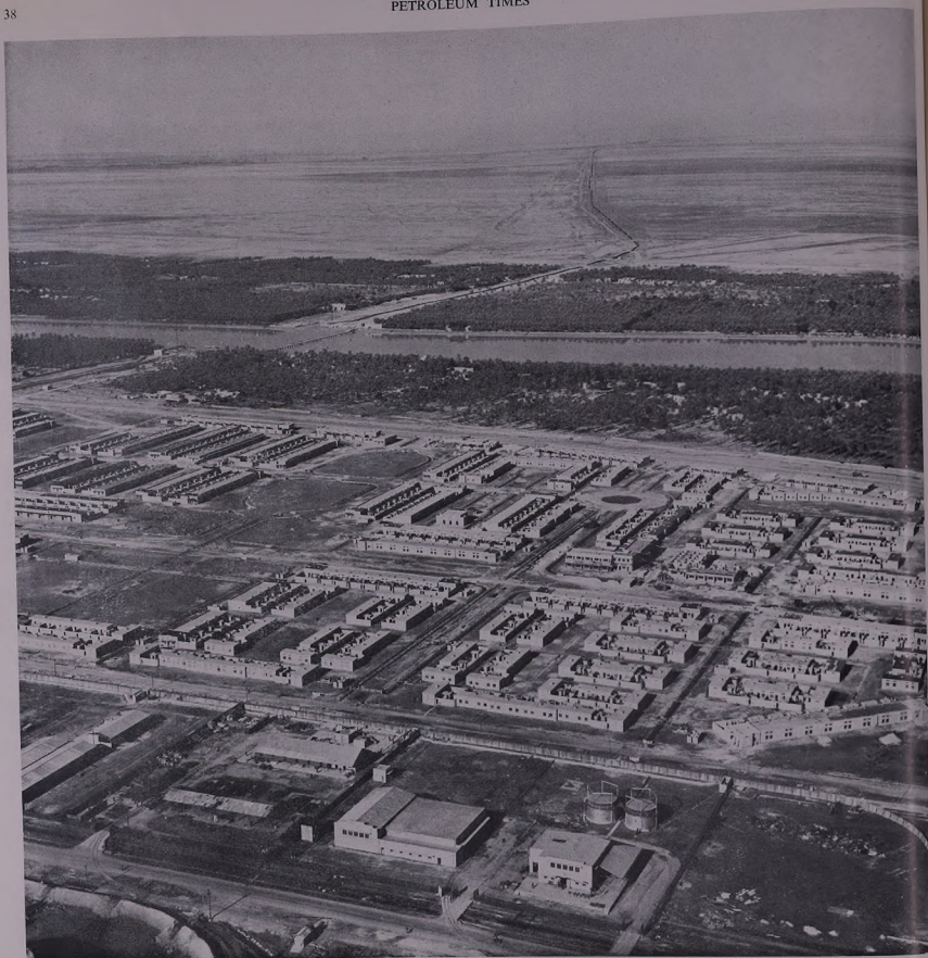
Air view of Farahabad housing estate for artisans
