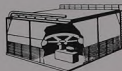
Fluor Fin-Fan cooling unit is especially indicated where space is limited and water is scarce.
