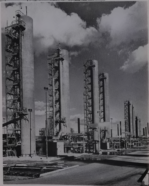
Super-fractionators for the preparation of aviation fuel
