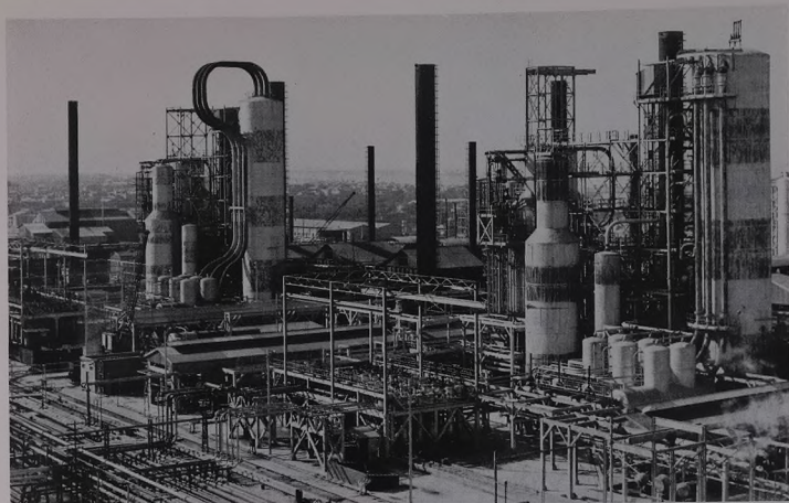
Two of the 3,000,000 gallons per day distillation units
