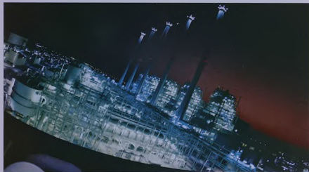
AL-KHOBAR Plant-Second Phase
