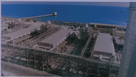
A general View of the AL-KHOBAR Plant
