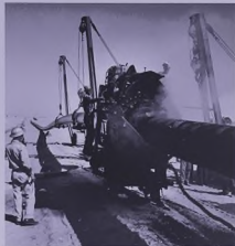
The new Khursaniyah pipeline, before it is buried, is tarred and wrapped to guard against corrosion.
