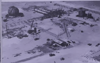
New construction for Khursaniyah production.
