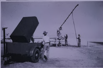
Bafco petroleum engineering crew running subsurface pressure recorder.
