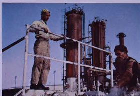
Bahman Operator Hady Hassan directs pipe fitter.
