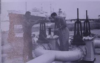
Fao Terminal: loading manifold
