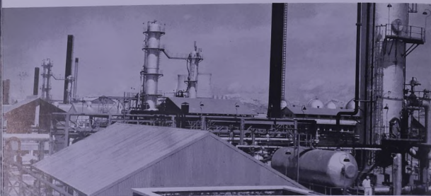
Kirkuk Process Plant: capable of stabilising 25 million tons of oil annually
