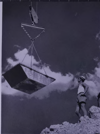
Construction at Dokan Dam: lowering a load of concrete
