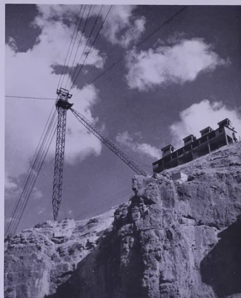
Preliminary work at Dokan; (above) the wall into which one end of the 385-foot high dam will be keyed, (left) a temporary cable bridge spans the gorge
