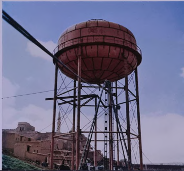
New water tank at Mosul
