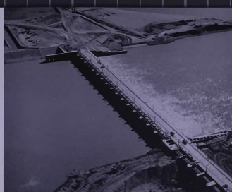
The waters of the Tigris flow through the barrage at Samarra – part of a ID16 million flood-control and irrigation scheme opened in 1956 by HM King Faisal II
