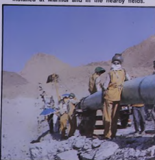
Construction of the gas pipeline from Yibal to al-Ghubrah.
