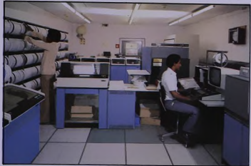
Inside the main computer centre at Mina al-Fahal.
