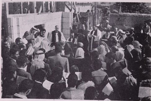
Service of the laying of the corner stone of the Church in Zerka.
