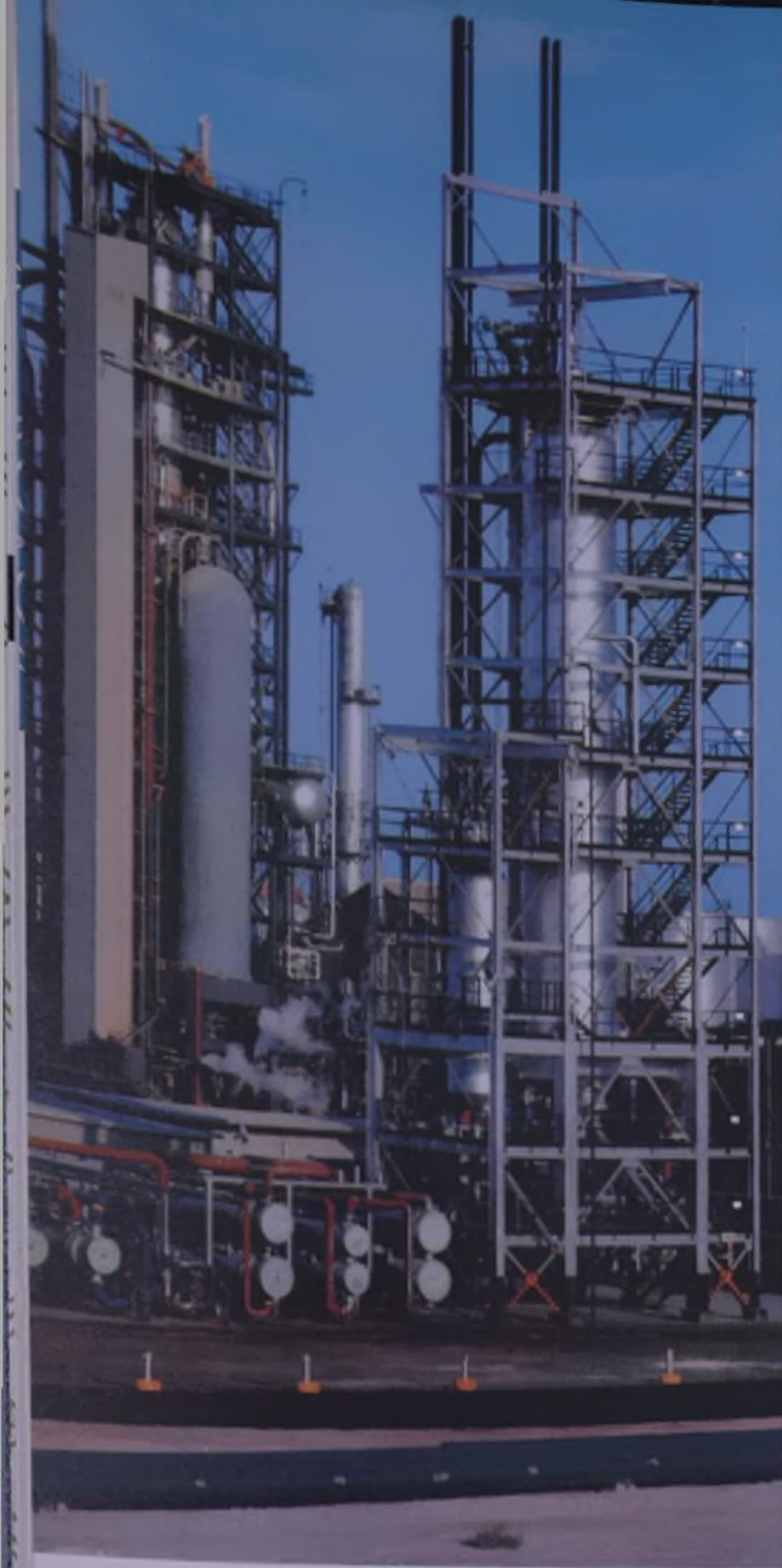
The catalytic desulfurizer (right) is the largest addition to the Ras Tanura refinery since the hydroformer (left).
