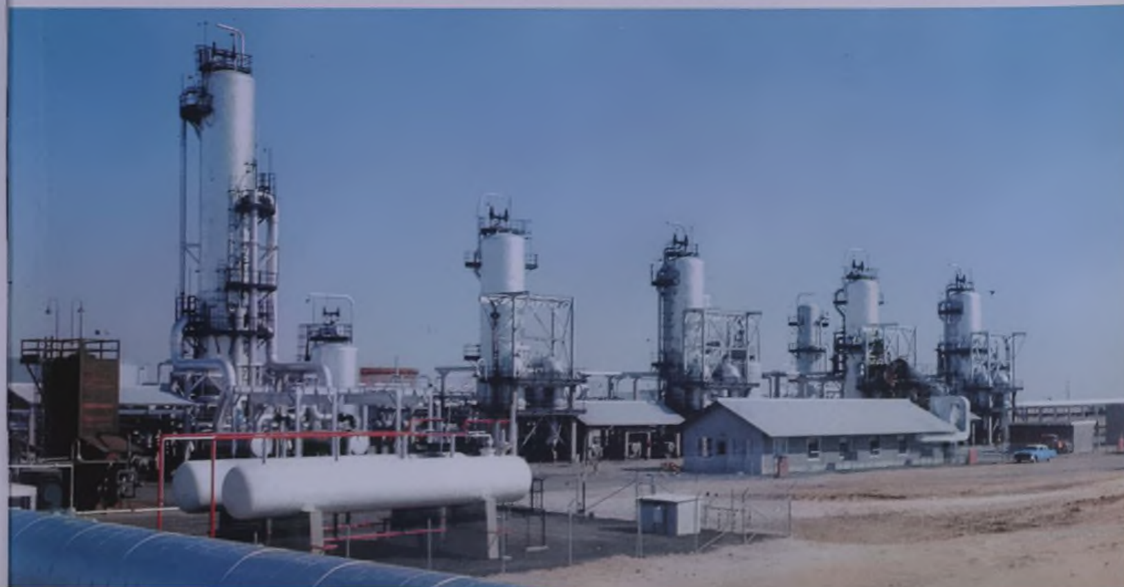
The new stabilizer column at Abqaiq, larger than the older columns, makes it possible to process more crude oil there.
