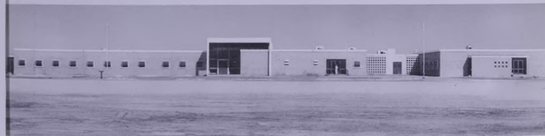
This new hospital-clinic at Ras Tanura contains the finest available medical equipment.
