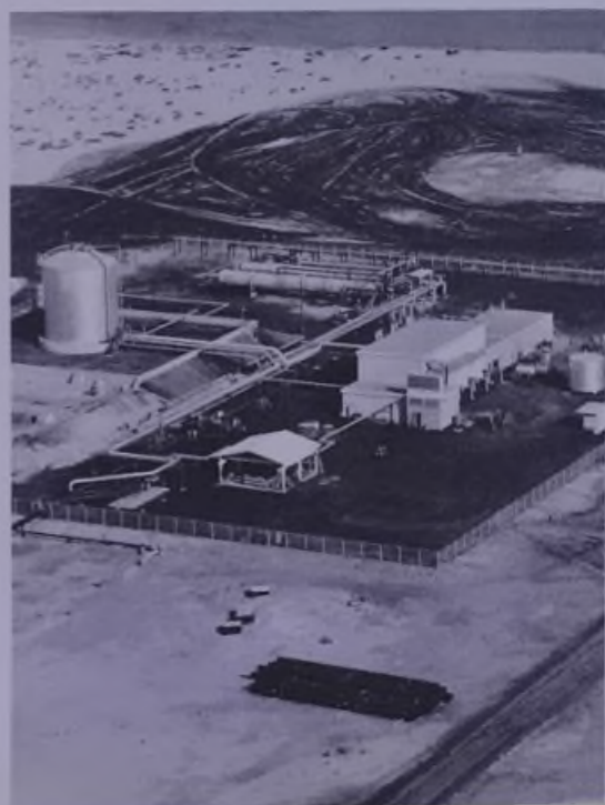
The Safaniya GOSP and pump station are being expanded to boost offshore producing capacity.
