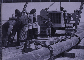
along the pipelines . . .
