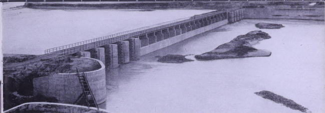
The Karkheh dam in Khuzistan
