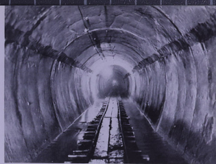
inside the Kührang tunnel
