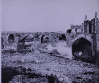
'Valerian's bridge' at Shushtar
