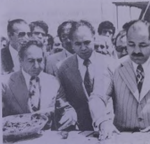
Mr. Taha Yasin Ramadan, RCC member, and Minister of Works and Housing laying the foundation stone of one of the housing projects in Baghdad.
