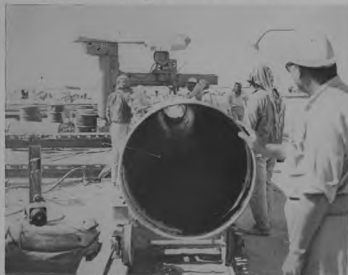
Pipe laying operations from al Raudhatain to Kuwait town, in progress
