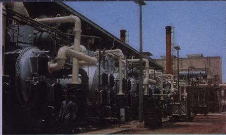
Only clean sea water is allowed for distillation. Marine life, herbs of foreign elements are removed by filters as in this photo
