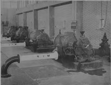
Water is pumped out from the underground huge reservoirs to the diverse points of distribution.
