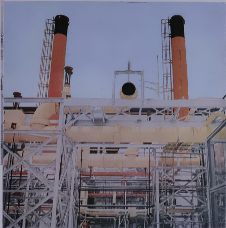
A distillery at the plant
