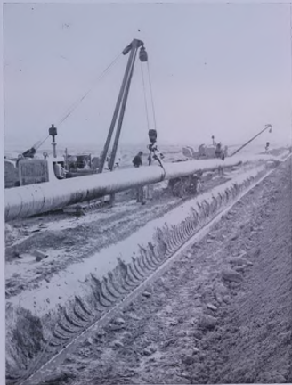
Laying of water pipelines feeding Kuwait
