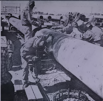
Work on the Raudhatain water pipeline
