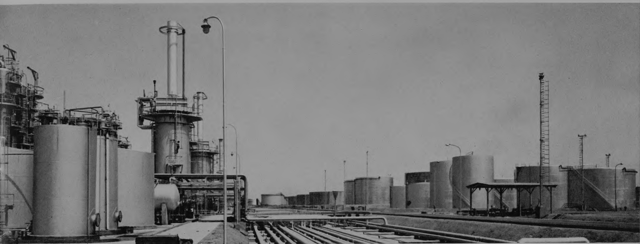
Partial view of the tank farms
