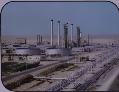
Mina al Ahmadi refinery
