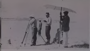
These men form a triangulation team who were seen at work near Kara Tepe Mountain. Based on data they collect, detailed maps will be drawn. From them, an alternate route designed to reduce the rate of climb and decrease tunnel requirements will be planned.
