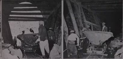
Construction in progress inside one of four tunnels being built along the Muş-Tatvan section. Whereas the longest will be 1,150 metres, this one nearing completion is 750 metres in length. In use is the "Belgian Method" of construction, whereby the top portion is dug out and covered with masonry before the bottom part is excavated. Debris is removed in carts pushed by hand along a narrow gauge, temporary track.
