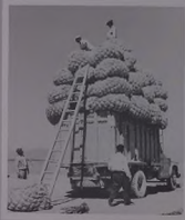
A short distance from Town of Shahpur, where surveying teams maintain an office, the party came upon a grain loading operation. When completed, the new Iran — Turkey link will be able to carry much larger and heavier loads more safely and for longer distances in both winter and summer.
