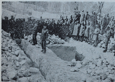
Corpsemen visit the construction of a public bath in a village during their training 4 months
