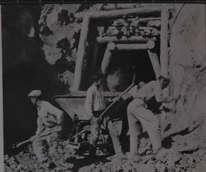
Many tunnels such as this one are under construction between Mus and Tatvan (Turkey) as part of the CENTO railway project.
