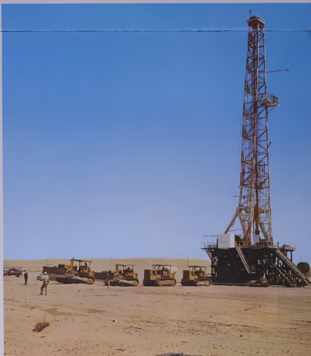
A rig move in progress.
