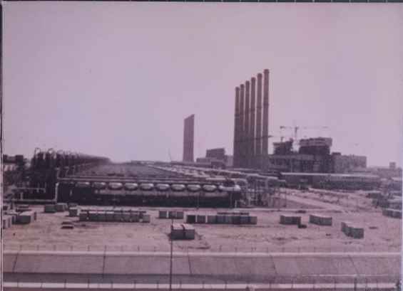
Desalination units. A general view of desalination and power plants.
