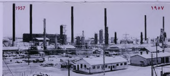
1936-37 Early refinery construction (right) and a view of the same area in 1957 (above). The first unit, a 10,000 BPSD crude still, came on stream in 1936. Construction continued and by the end of 1937 crude refining capacity had risen to 25,000 BPD.
