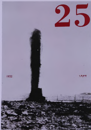
1932. On June 1st, at six o'clock in the morning, oil started flowing from Well No. 1 at a depth of 2,008 feet. The initial flow rate was 400 barrels an hour.
